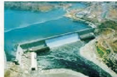
Dams and Reservoirs
